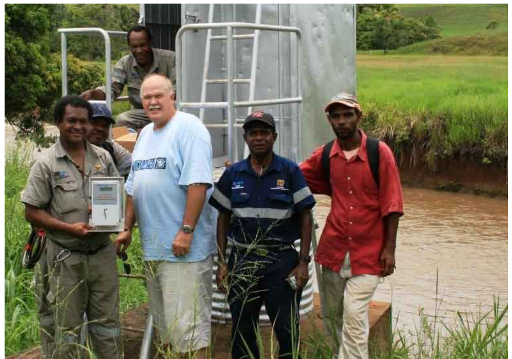
PNG's water 'oldies' and Marc Wilson, after a successful installation at Laloki.
